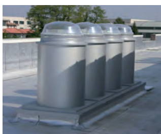
Bearing and square-based flashing with cylindrical flue and transom flashing (Massalengo school 2009)
